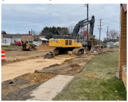
sion on the replacement storm sewer for the county drain to connect to the Scott Creek Drain. In addition left turn lanes will be added. curbs will installed and old sidewalks in disrepair will be fixed. Work is expected to continue throughout the summer. Please continue to follow posted detour signs.
